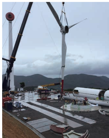
Windmill under demolition
