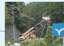
Electric power line replacement work in a mountainous region (Shiga)
