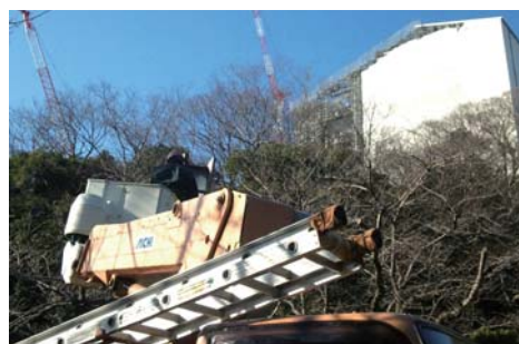
Cleaning at Himeji Castle, which is undergoing the renovation work
