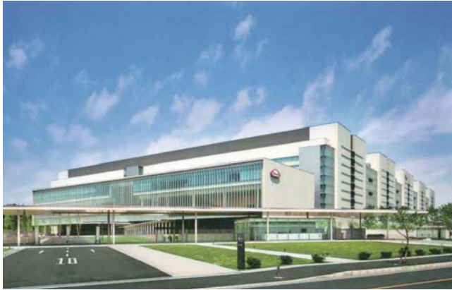
Electrical Shonan Research Center of Takeda Pharmaceutical Company Limited (Kanagawa)
