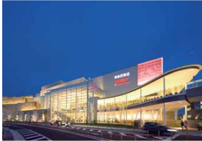
Electrical Hankyu Nishinomiya Gardens (Hyogo): Commercial complex
