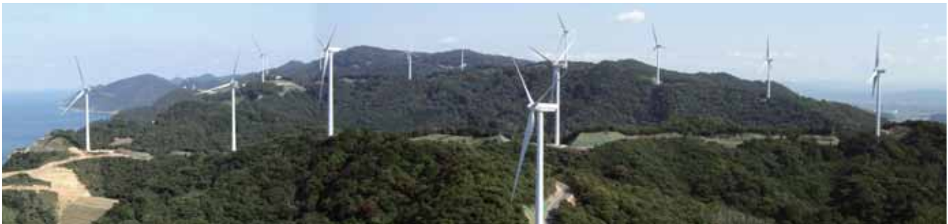
Shin Izumo Wind Power Plant consists of 26 wind turbine generators, each capable of generating 3,000 kW.
