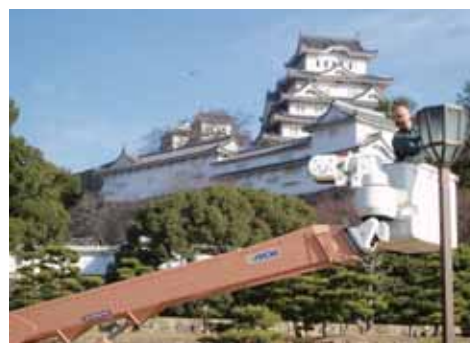
Clean-up activities at Himeji Castle
