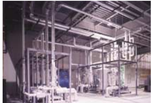
Environmental Management Facilities Toyoset Komagane Plant (Nagano)
