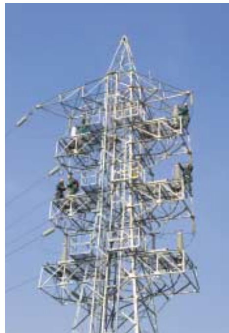
Electric Power & Others Transference work of existing transmission lines (Osaka)
