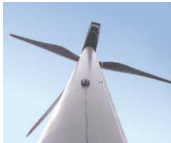
The robot climbs the exterior wall of a wind power generation tower.
