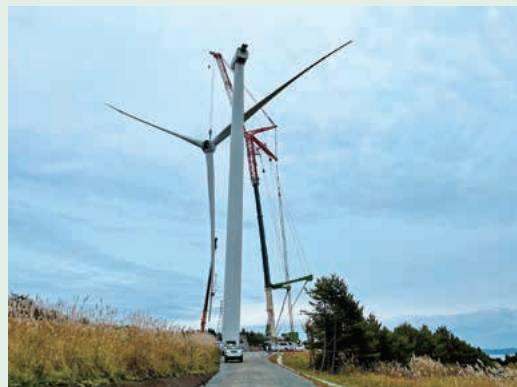
Hoisting the blade with a large crane
