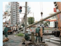
Rebuilding a broken power pole (Osaka)
