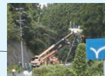
Electric power line replacement work in a mountainous region (Shiga)
